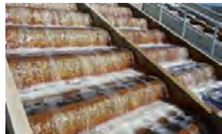
Station de pompage des CASCADES (Seychelles) / Water pumping plant of CASCADES (Seychelles)
