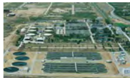
Station de pompage de CHOTRANA (Tunisie) / Pumping station of CHOTRANA (Tunisia)
